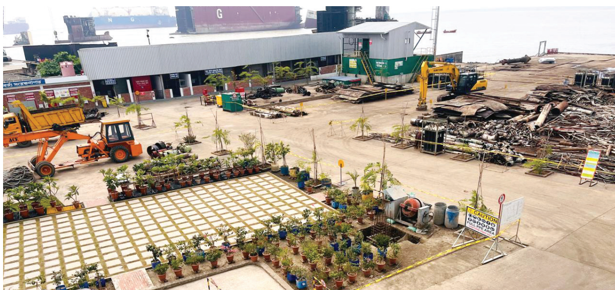
An OBPLC financed Steel Mill
